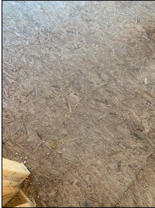
26. Subfloor - OSB (Oriented Strand Board)
