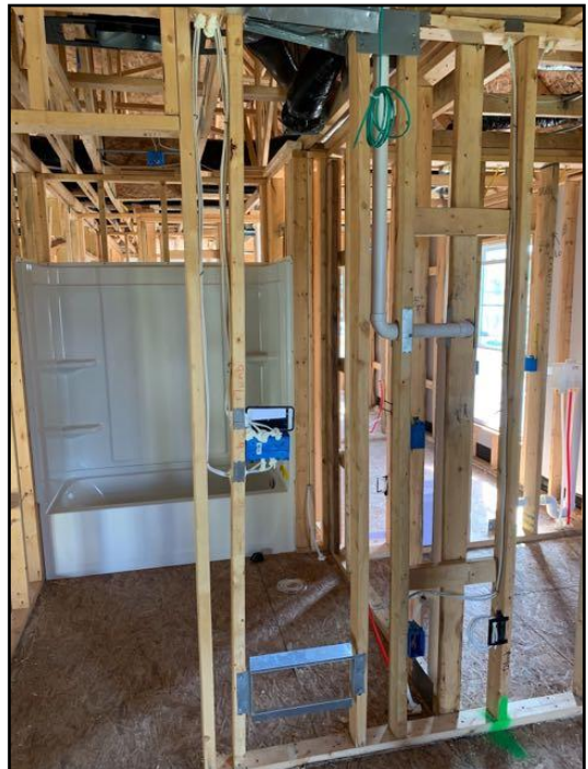
46. Leaning, bowing, buckling
