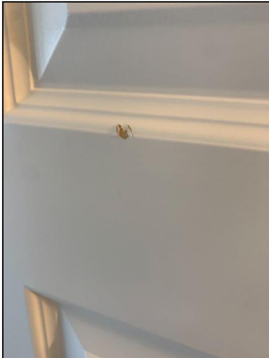
109. The door slab has cosmetic defects in the...
