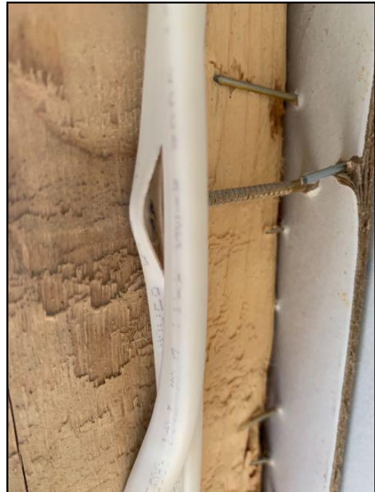
67. Poor nailing
