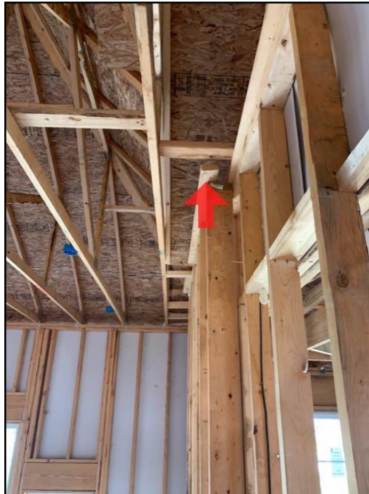
54. Un-flush Studs within the framing system ca...
