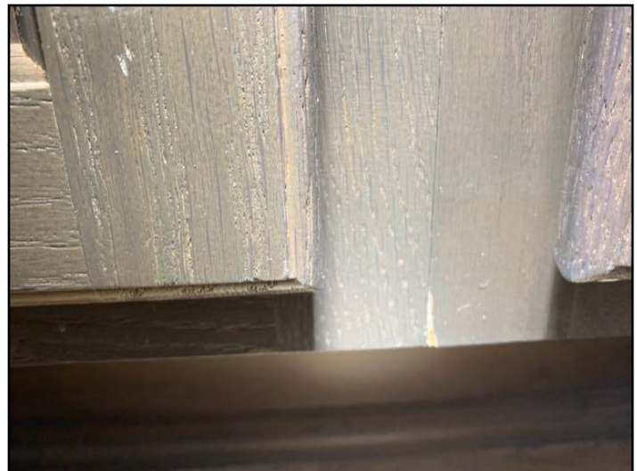
119. The cabinets have cosmetic defects in the...
