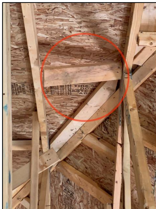
58. Truss installation have both temporary and...
