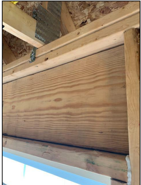
94. The caulking sealing the void between the...
