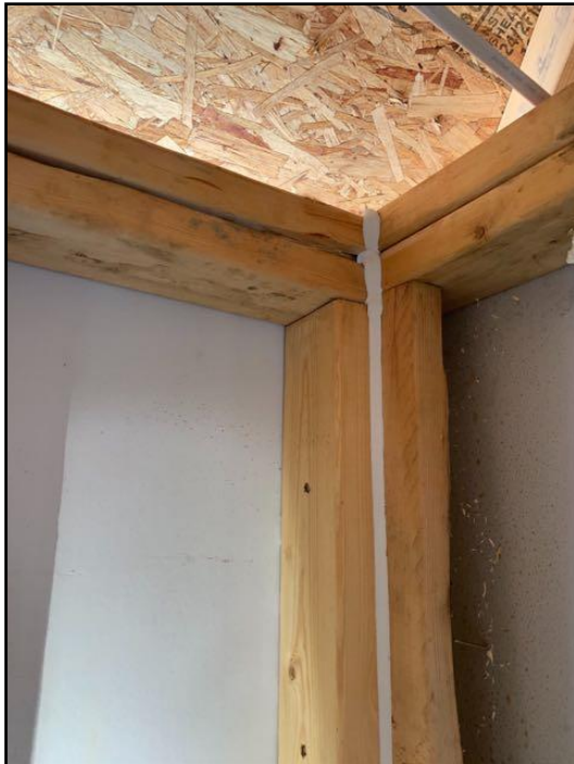
93. The caulking sealing the void between the...
