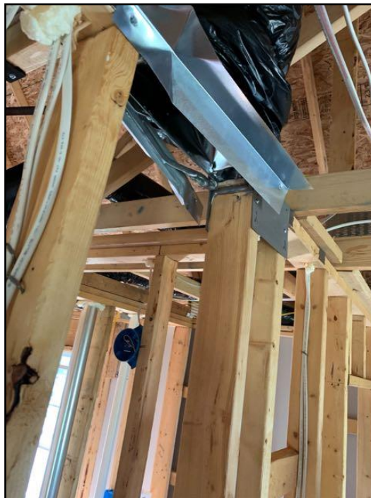
84. Disconnected ducts
