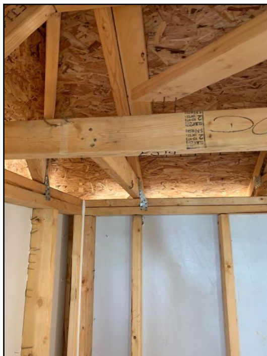
57. Truss installation have both temporary and...
