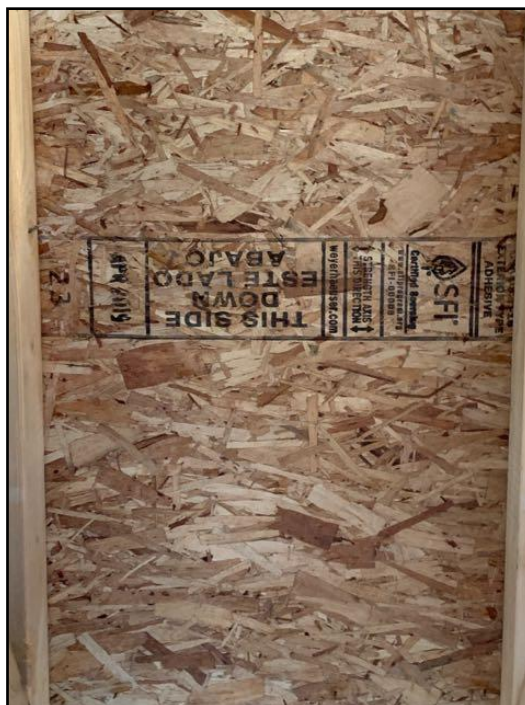
28. Oriented Strand Board (OSB) sheathing
