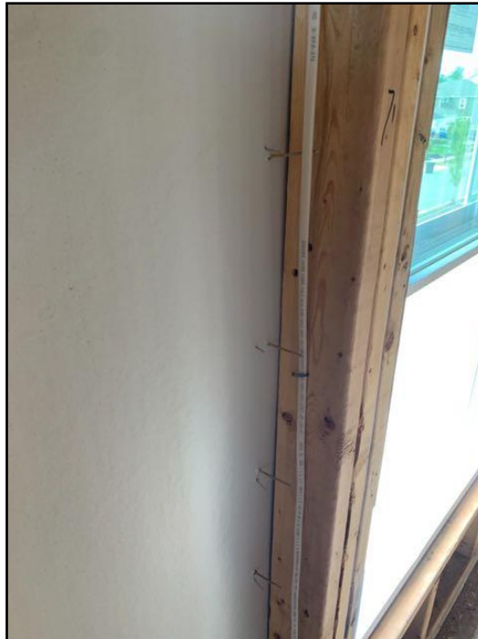
41. Poor nailing
