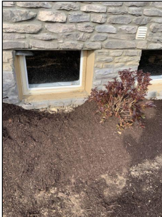
23. A window well is the area outside a...
