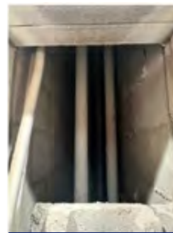
Non ACM Pipe Insulation
