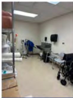
Non ACM Wall System
