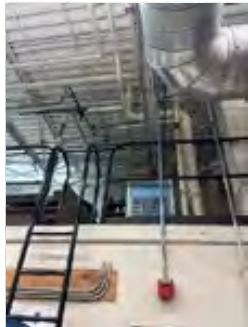
Non ACM Pipe Insulation
