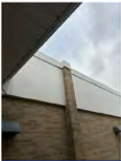
Non ACM Exterior Panels
