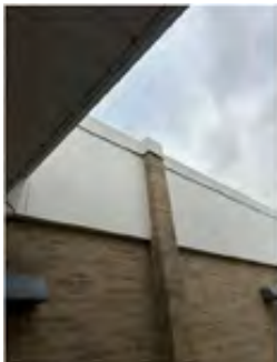
Non ACM Exterior Panels
