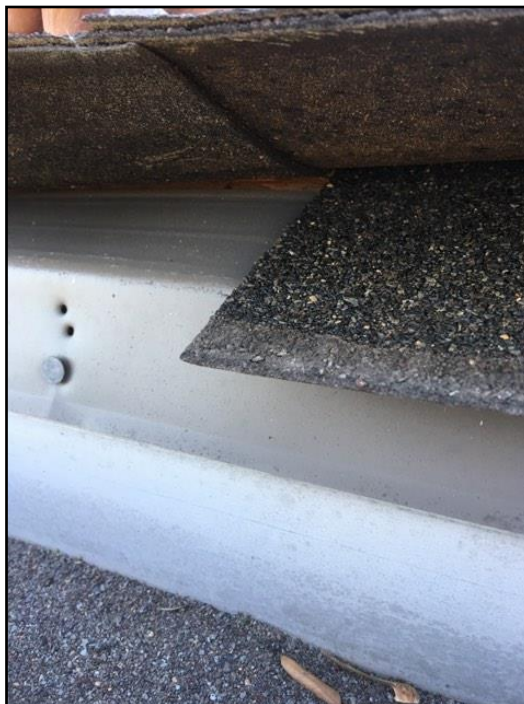
5. Ice and Water shield is a critical componen...
